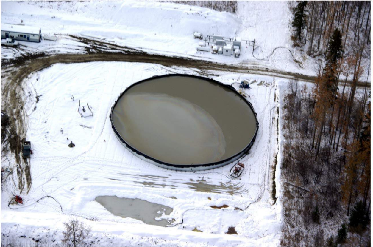
Frac Water Tank 138' Diameter x 7' 4" High Capacity: 3,076 m 3 Fort St. John, B.C.
