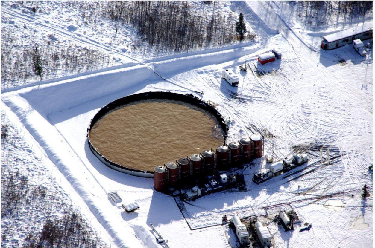
Frac Water Tank 138' Diameter x 11' High Capacity: 4,614 m 3 Farrell Creek, B.C.
